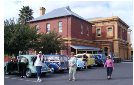
Werris Creek Railway Station
